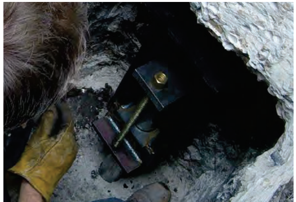
Figure 2.56 Place bracket assembly onto last driven pier tube
