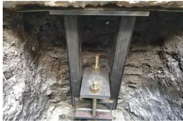
Figure 2.58 Completed concentric pier installation
